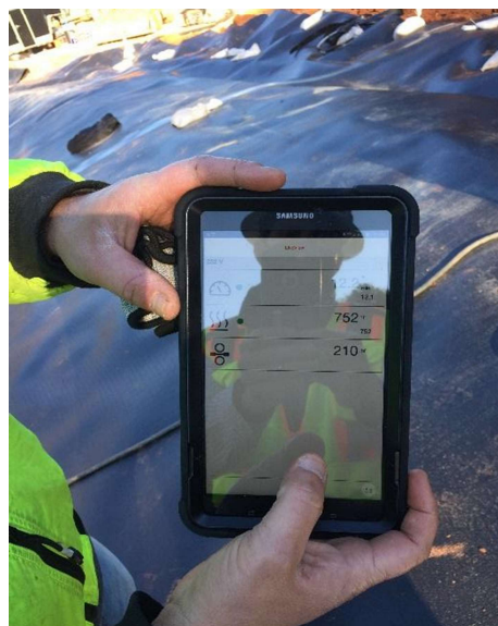
Figure 5: Tablet PC connected to the Data Acquisition Welding machine displaying seaming parameters.
