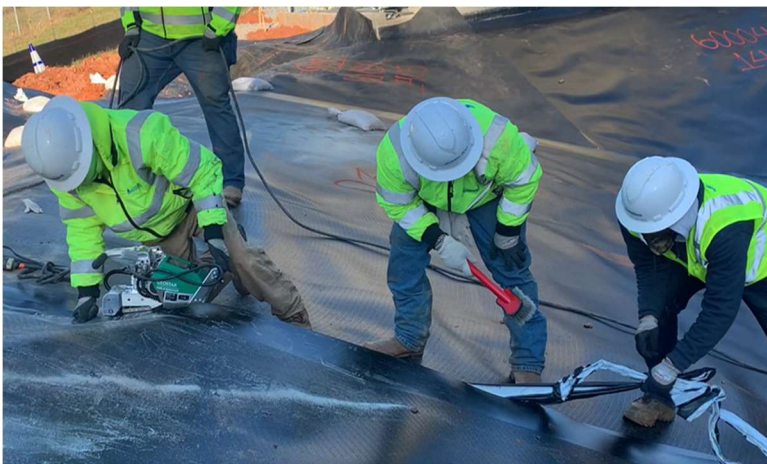
Figure 3: Geomembrane seaming in progress – tape removal (right) ahead of seaming (left).
