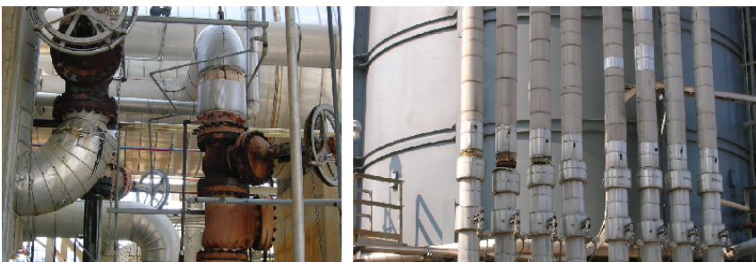
Fig. 3: Poor or unfinished installation, mechanical damage and signs of abuse during access are typical of aged insulation and jacketing in refineries and chemical plants. Evidence indicating a lack of CUI inspection and lack of maintenance on these easy-access feeder runs is clearly visible.
