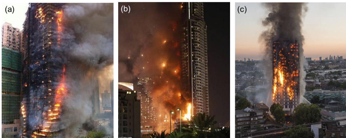
Fig. 1. (a) Shanghai Jing'an fire in 2010, (b) Dubai Address Tower fire in 2015, (c) London Grenfell Tower fire in 2017.
