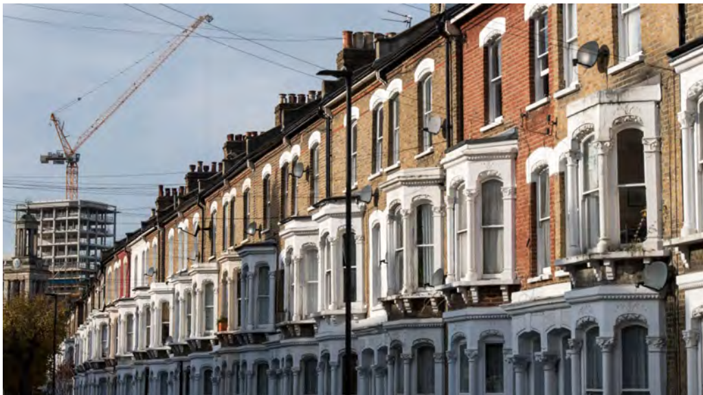
Building surveyors were for many years employed directly by the developers whose work they needed to approve. BLOOMBERG
