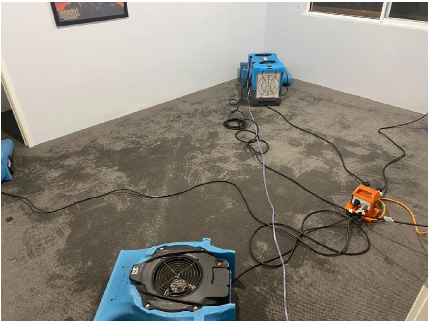
📷 The Iplex piping issue. It has ruined carpets and wrecked furniture. Credit: Supplied/Supplied
