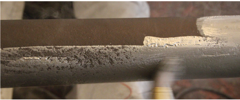
Fig. 10: The hot-spread epoxy phenolic coating was brush-applied to hot steel pipes.
