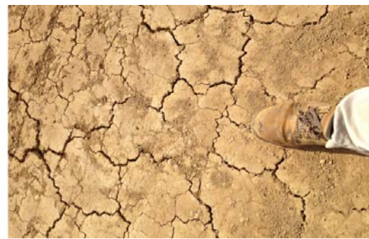
Figure 10. Unacceptable desiccation of clay sub grade [Scheirs]
