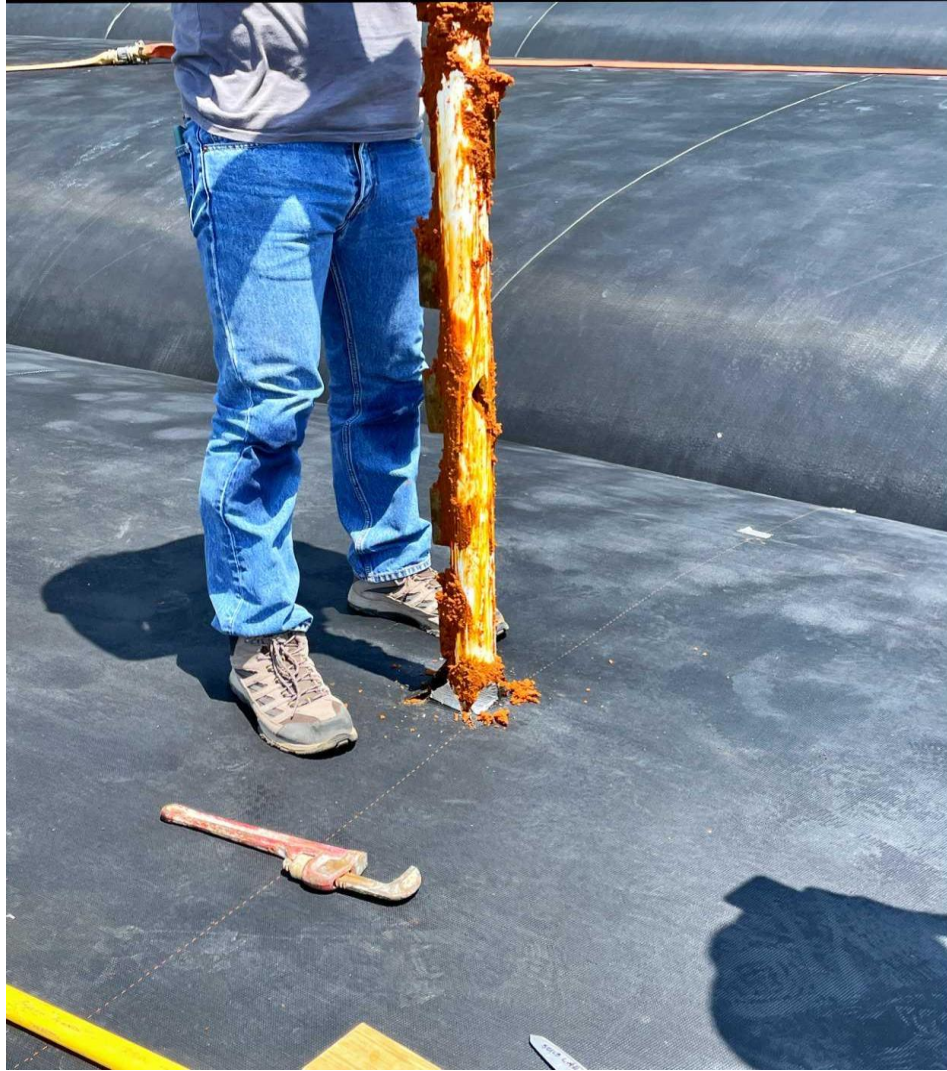
Figure 13: Removal of Sludge Sampler (Source: Tyson 2022)
