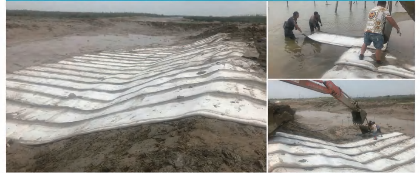
Jiangsu Yancheng Dongtai Luneng revetment project
