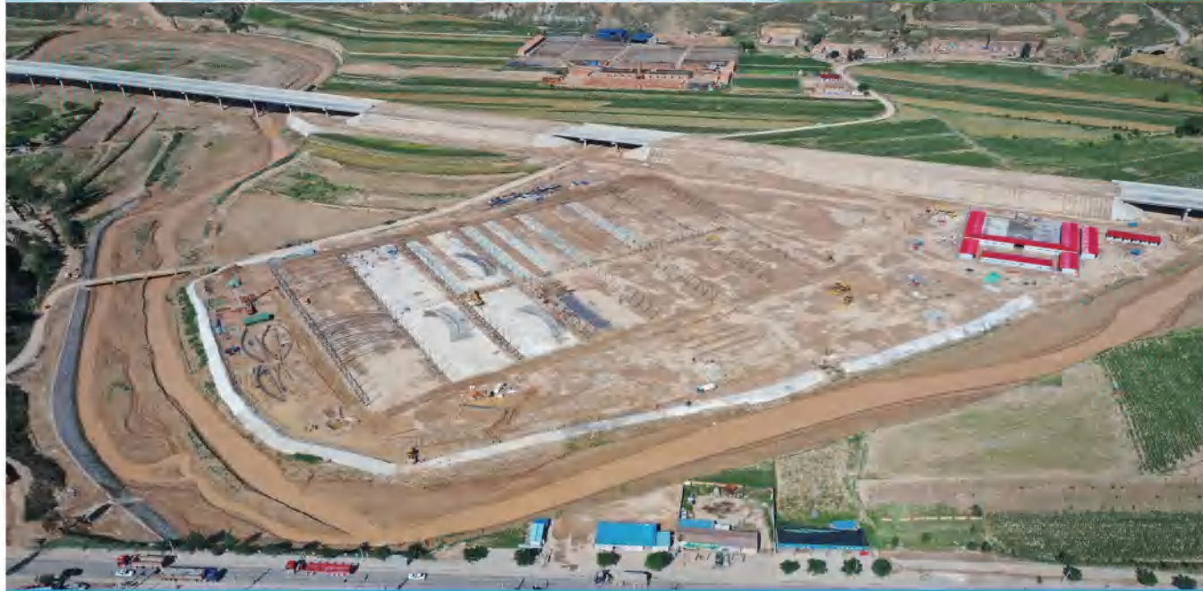
Mineral washing pool
