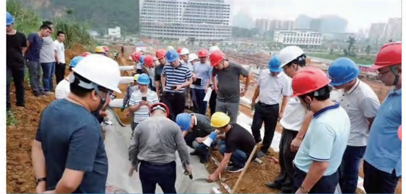
Construction site training meeting
