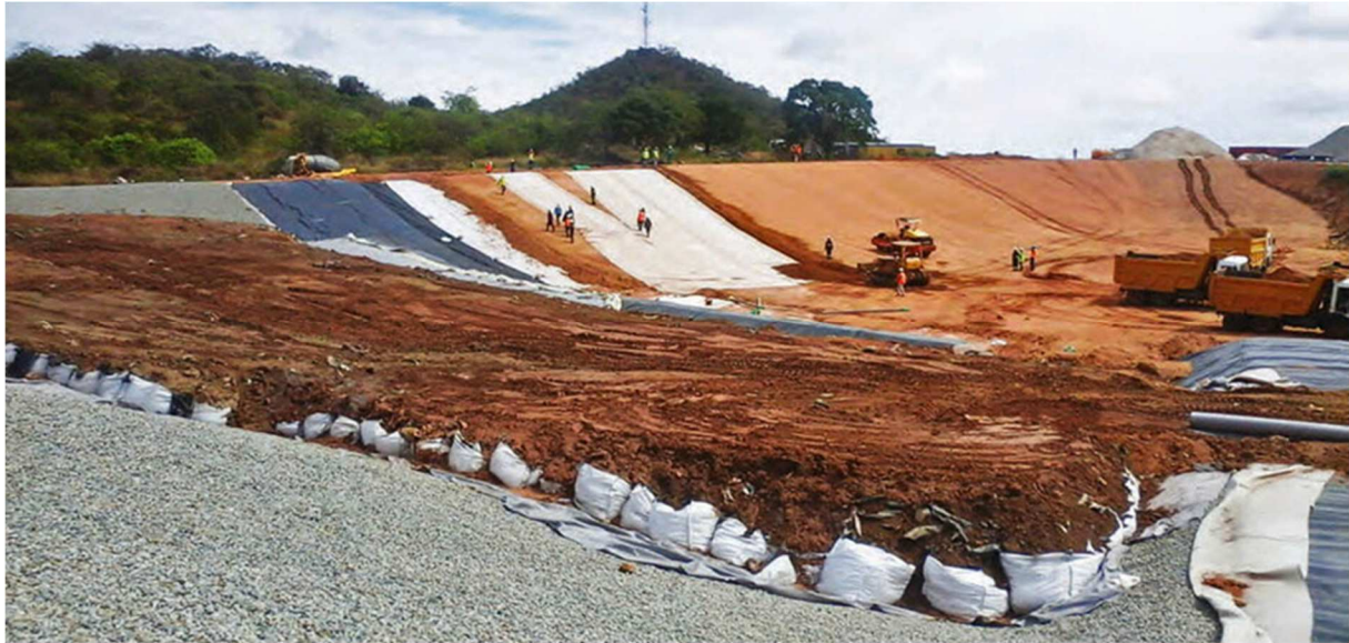
Figure 8: Installation of the base lining system [39]
