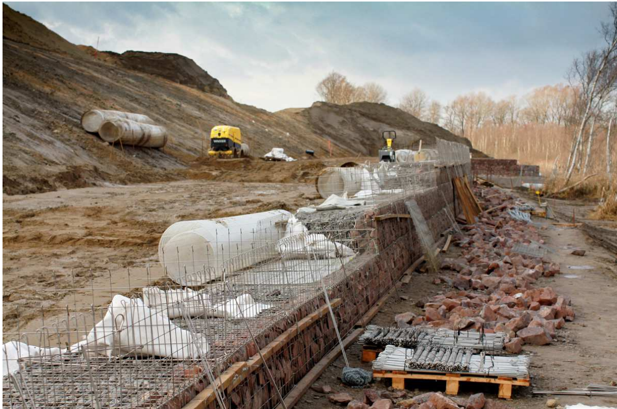
Figure 11: MSE berm around the perimeter of the Hanover landfill, Germany
