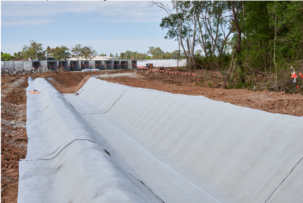
Tiltex B 5 M Wide roll installation at a major Sydney channel lining project.
