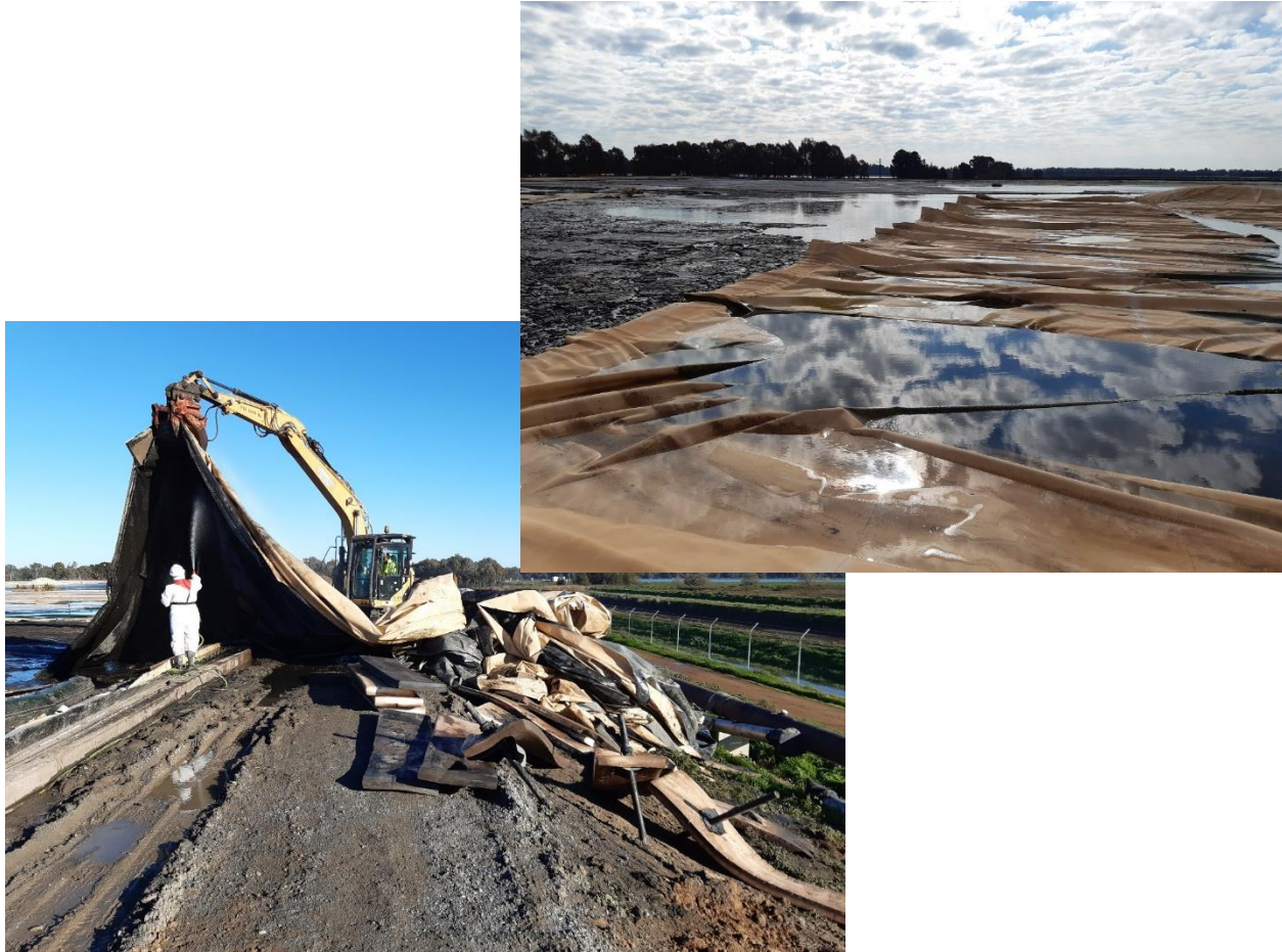
Photos above: Fabtech Undertaking Cover removal
