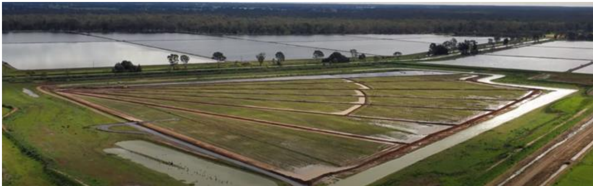
Photos above: Fabtech Undertaking Desludging and Descumming Works
