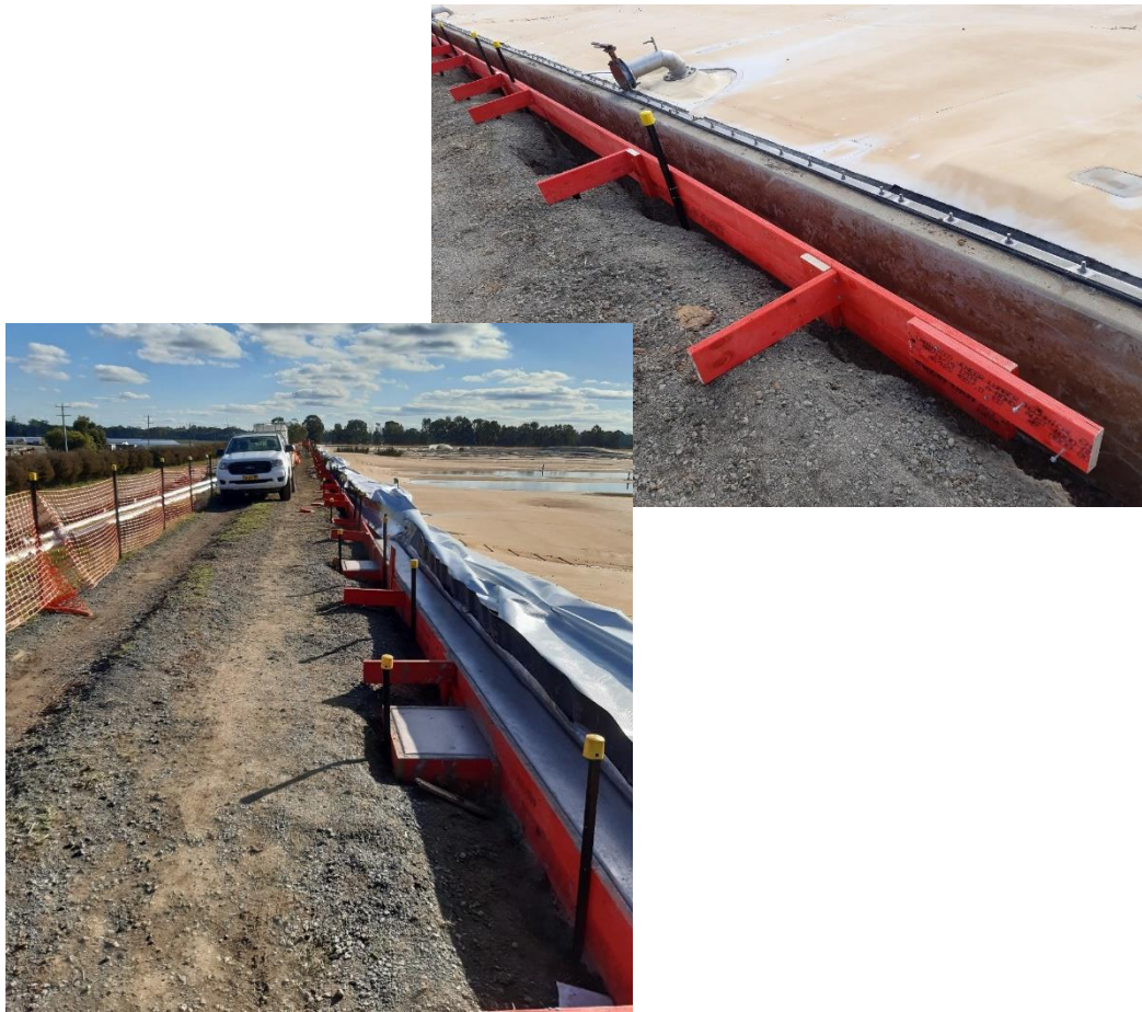
Photos above: Fabtech Undertaking Concrete Ring Beam reworks and replacement
