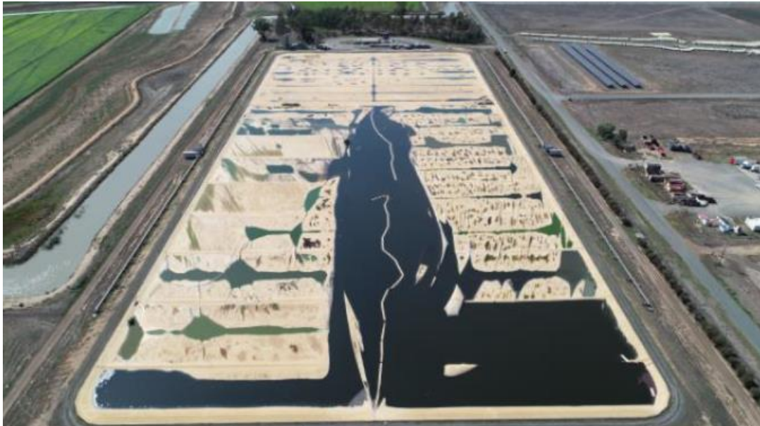
Photos above: The tear in the cover is significant, measuring over 200m in length - photo dated 2020
