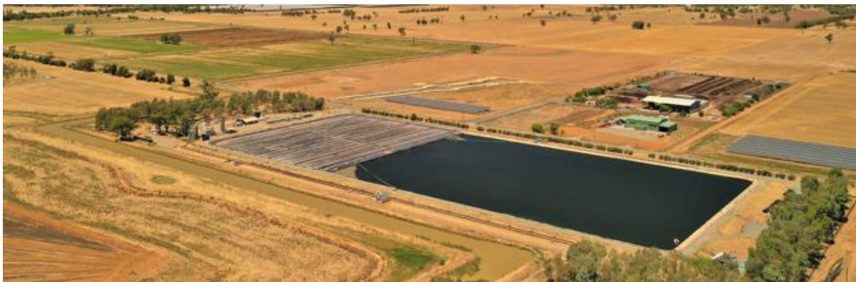
Photos above: Fabtech Undertaking Cover replacement stage 1 (Reactor Zone)
