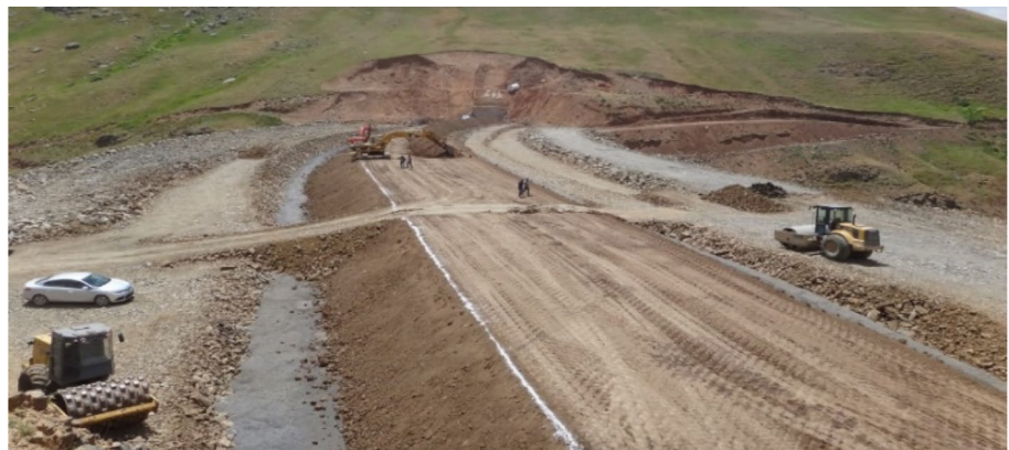
Fig. 14 Impervious clay supported by GCLs at Morgedik Dam (DSI 2015)
