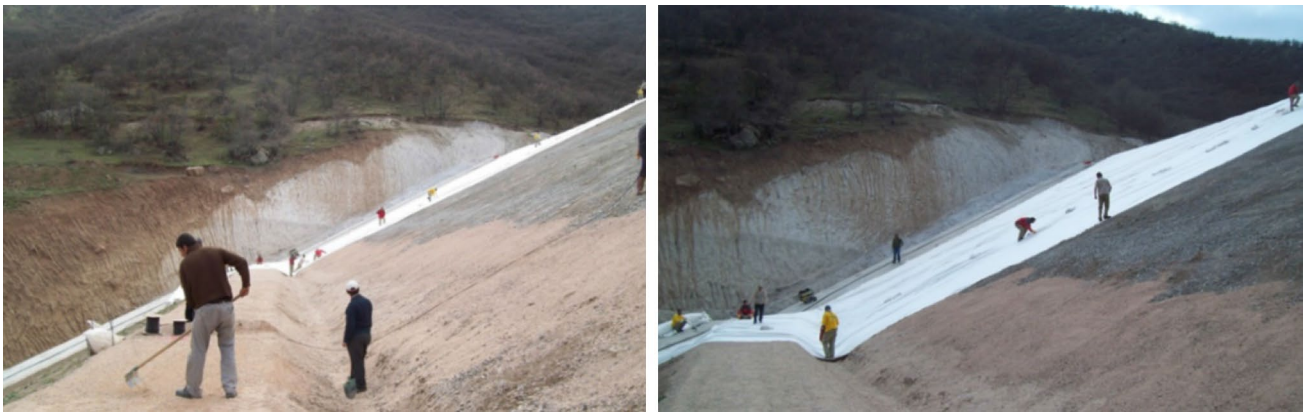
Fig. 11 Geomembrane sealing systems on the upstream face of Yedikapı Dam
