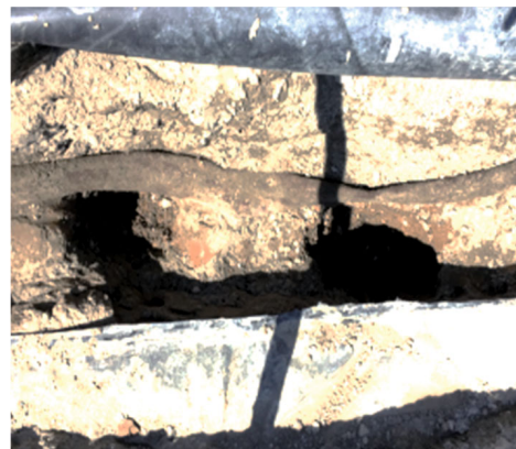
Sinkholes formed in loam
