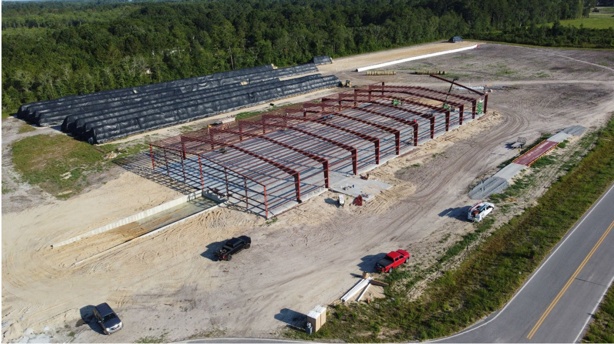
Steel frame of the building being erected June 20, 2022.
