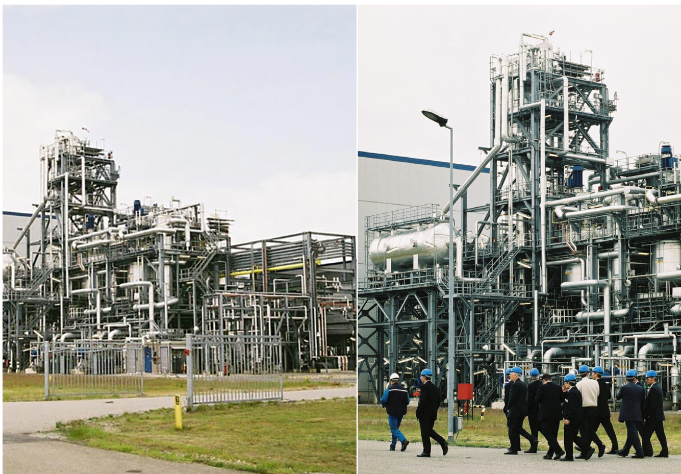
Figure 10. LyondellBasell Polybutene Manufacturing plant, Moerdijk, The Netherlands
