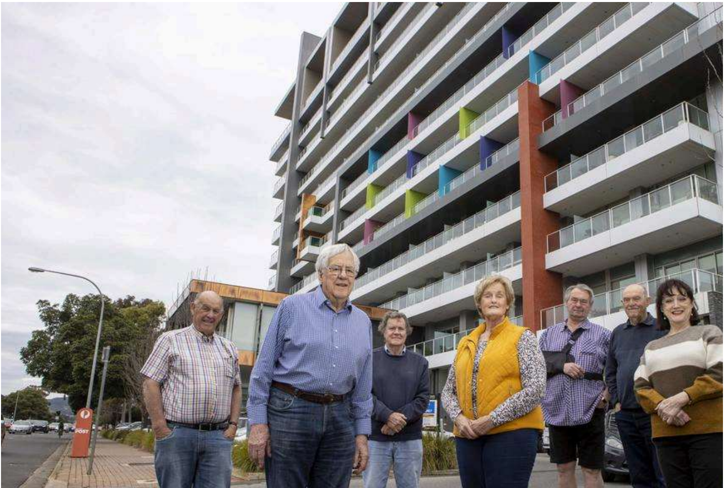
Residents of the Air Apartments who have concerns about flammable cladding on the apartment building. Picture: NCA NewsWire / Kelly Barnes
