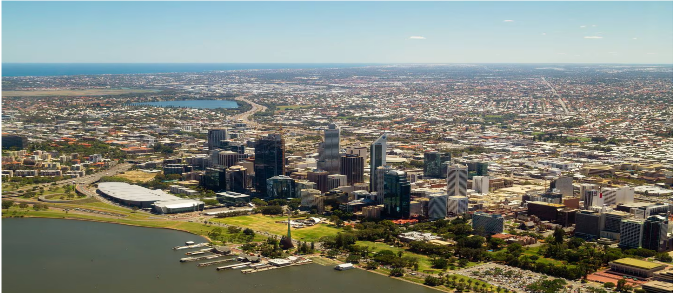
Perth, where hundreds of homes' water pipes have leaked. These pipes were mainly installed from 2017 to 2022.
