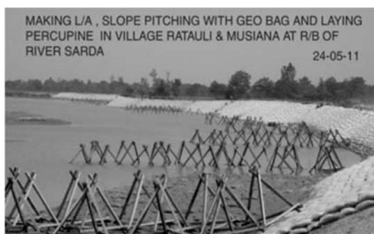
Fig.13: Use of sand bags (geotainers) in erosion protection at River Sarada
