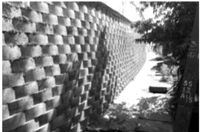
**Fig. 4:** The Block faced wall at Eluru
