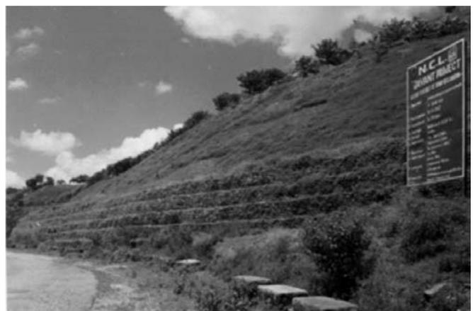
**Fig. 11:** Erosion control by Jute Geotextile in mine dumps
