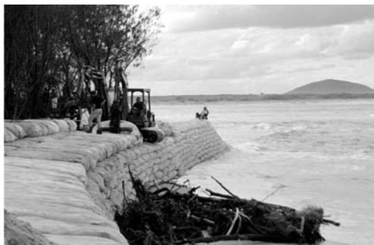
Fig. 12: Control of Coastal Erosion by Geotainers (Photo Courtesy : M.Venkataraman)
