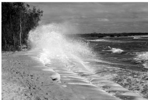
Fig. 14: Indigenous geotube for coastal erosion
