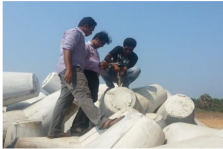
Fig. 1. Tetrapod at Uppunda shore and Non-Destructive Testing by using Rebound hammer.
