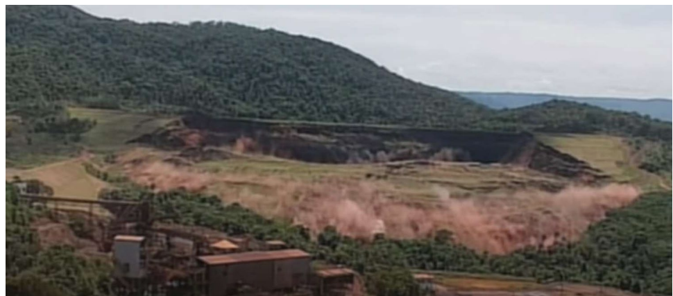
Fig. 4 After a few seconds, the failure propagated throughout the Feijão Dam I (modified from public images first shown on TV by Globo)
