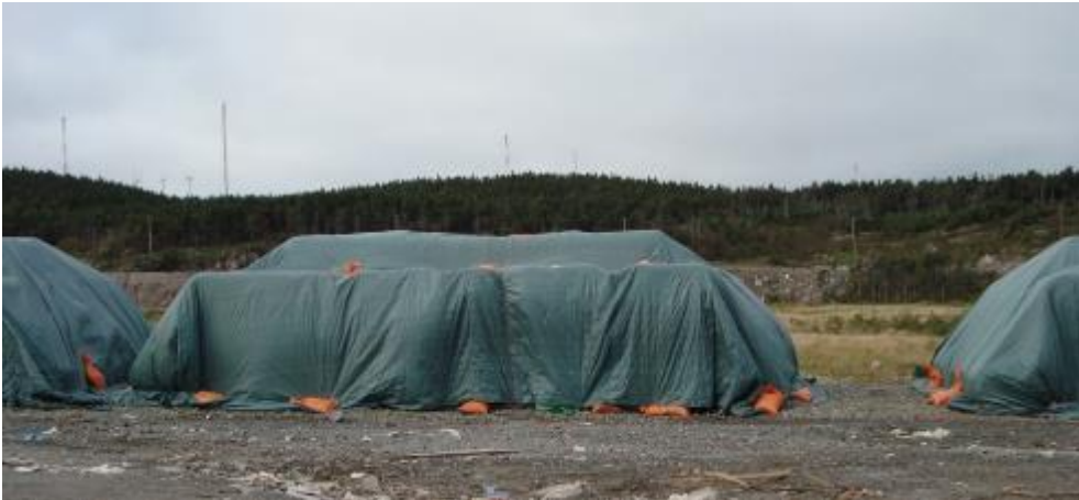
Figure 2.2: Tarpaulin installed on top of a pile of GBR-C for site storage (photo courtesy Terrafix Geosynthetics)
