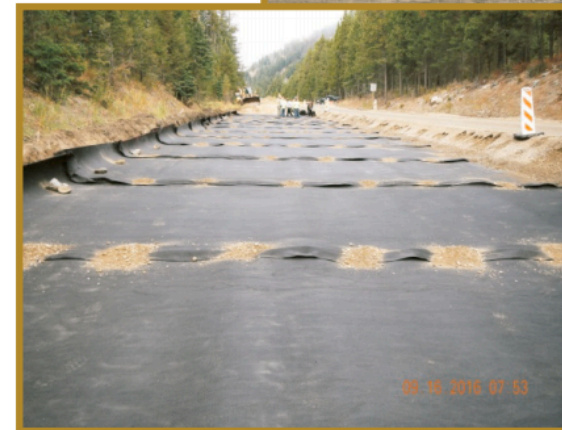
SSDL traversing both lanes and ready for base course application
