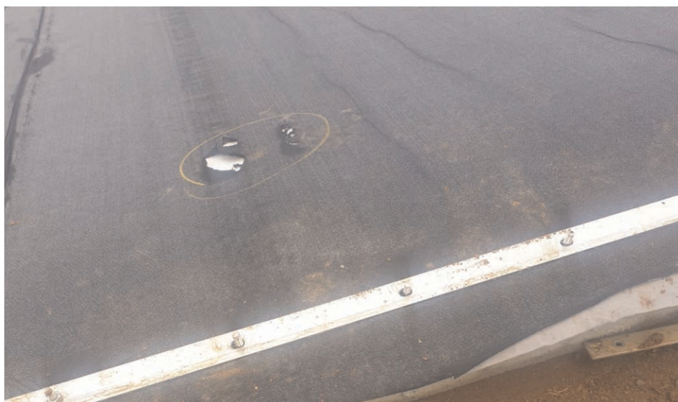
Figure 5. Holes in a conductive composite made by workers walking on it. These required patching to ensure adequate conductivity.
