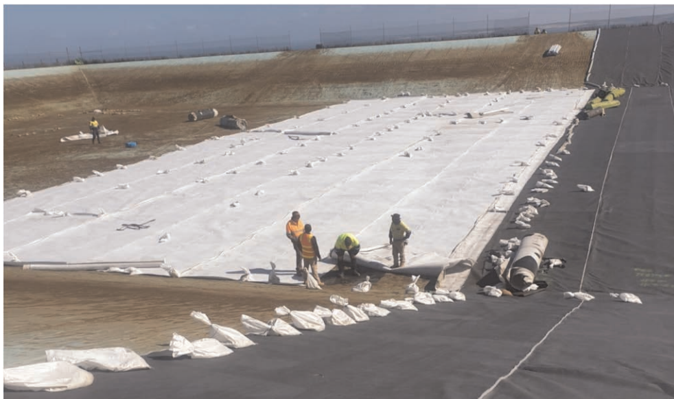
Figure 3. A reservoir with the old discoloured fPP liner being used as a secondary liner. The white material on the floor is a drainage geocomposite and the black material on the slopes and the floor is a conductive non-woven geotextile with a unit mass of about 350 gsm.
