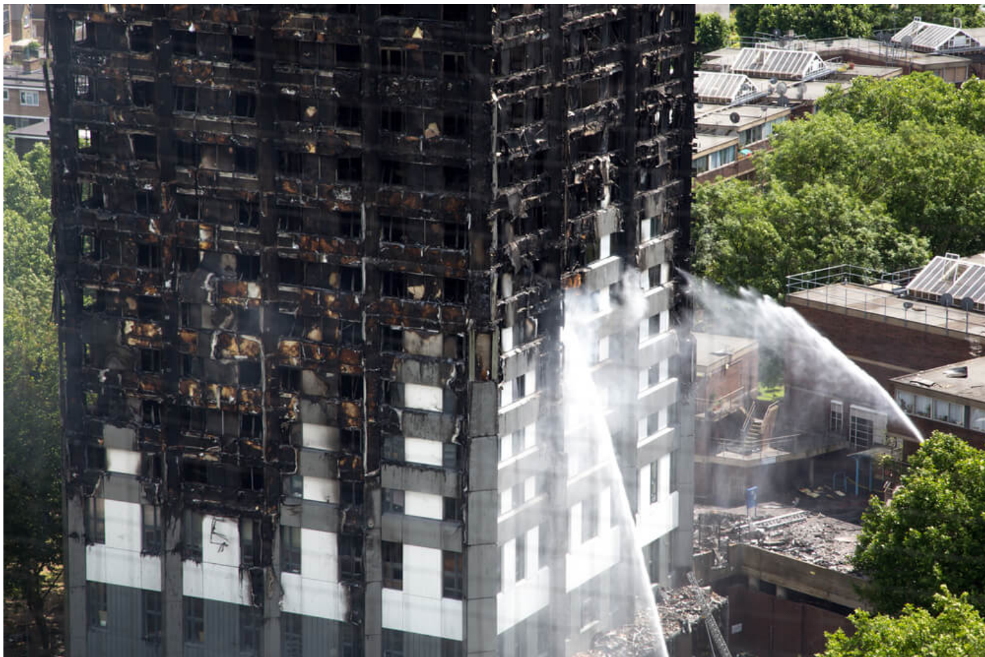
2017 fire at Grenfell Tower in North Kensington, West London
