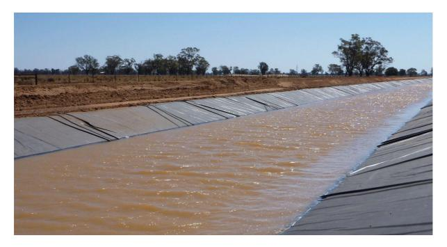
Without getting into specific on the failures being experienced there are general rules that apply for using flexible liners in canals and channels.
