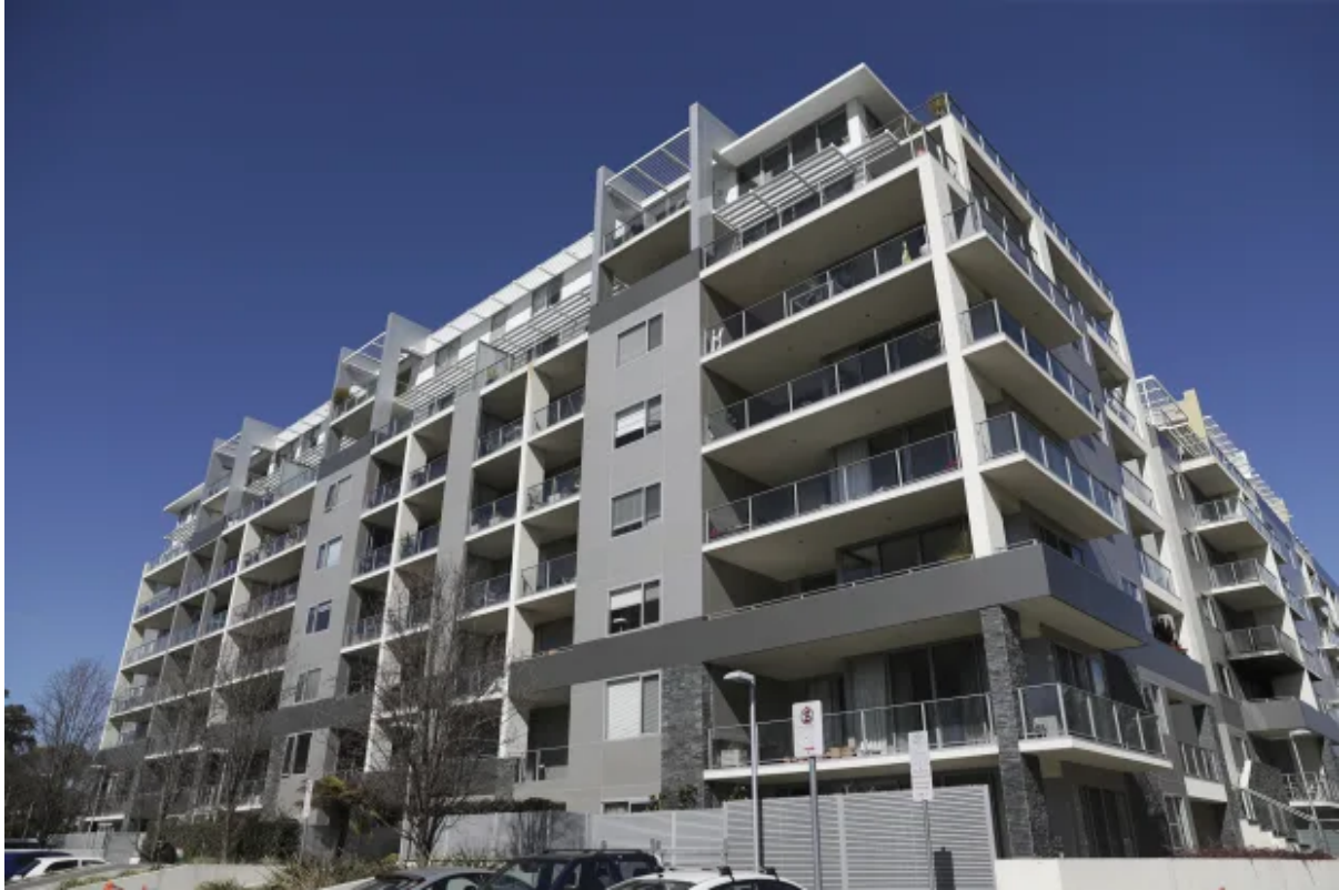
Glebe Park Apartments in Canberra. Alex Ellinghausen
