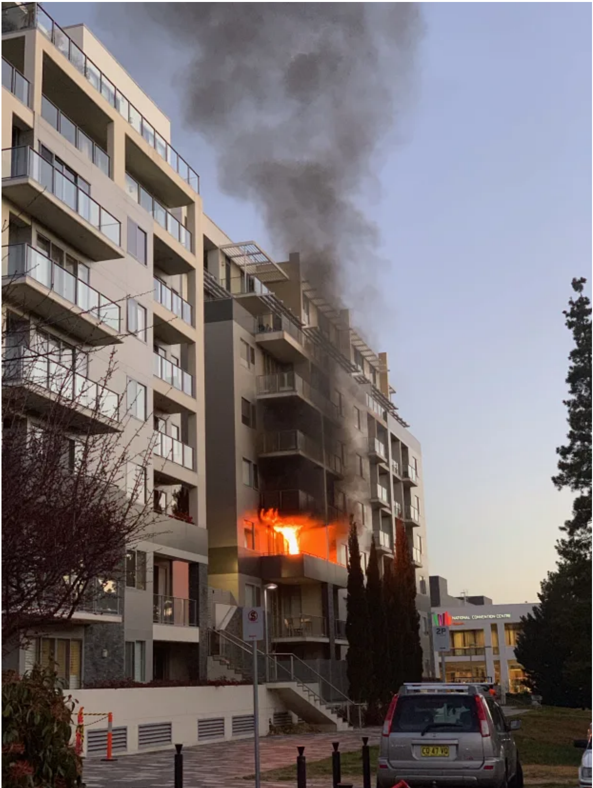
The balcony fire at the Glebe Park Apartments in Canberra on August 7, 2019. Nine
