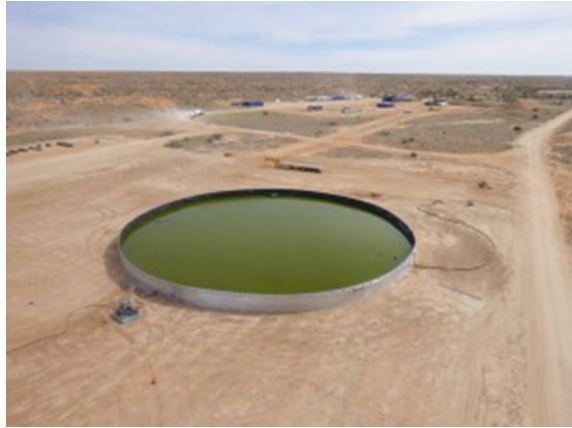
Fig. 16.3 Relocatable above ground water storage tank
