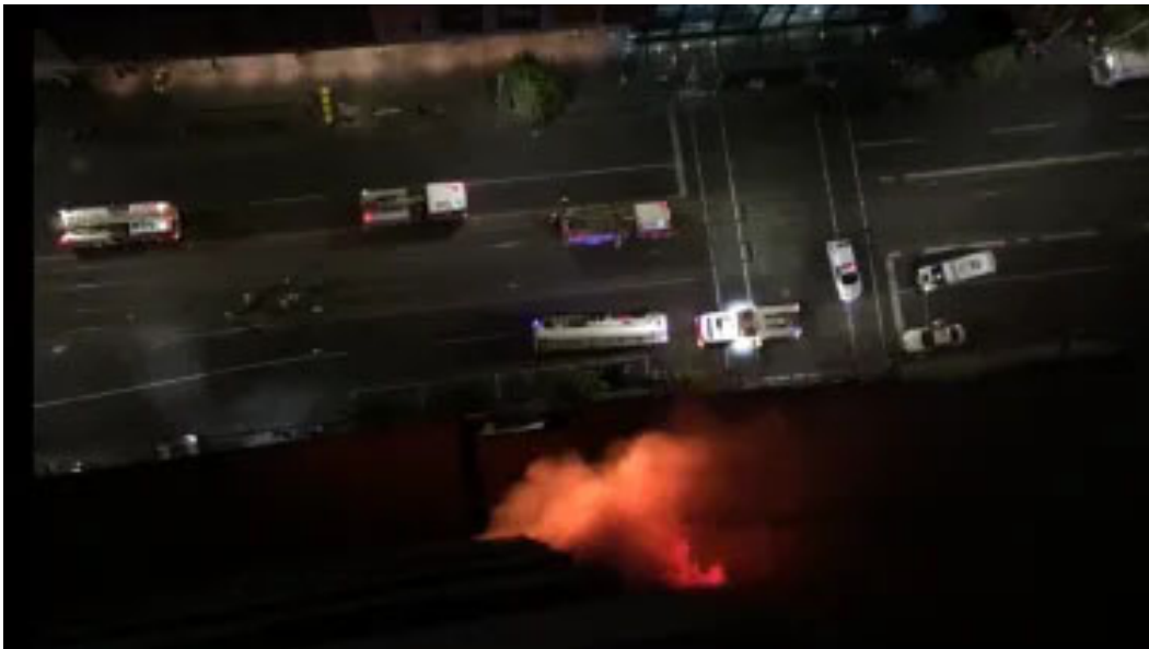
A resident's view of the Neo 200 cladding fire in Spencer Street in 2019. The public will pay some of the repair bill.
