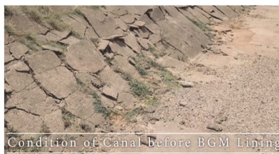
Figure 2. Original condition of canal stretch.
