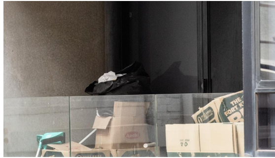
📷 Balconies at the Neo200 apartment building were stocked with flammable material. Picture: Jason Edwards
