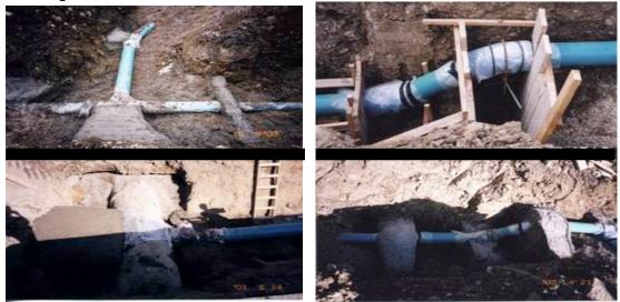
learned that inspectors view concrete as very cheap and repairs very expensive, so thrust blocks and concrete forms tend to be sized conservatively as shown in Fig 10, above.
