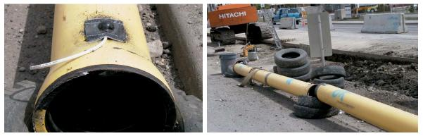
To prevent scratches from occurring during installation, the pipe is moved with cloth straps, not chains; and bedded in 150mm of sand or "pea gravel" (smooth rock, 10-15mm) followed by an additional 150mm to cover the top of pipe. Only then is granular fill such as gravel or native soil backfill permitted. The electrical continuity of the pipe, and current flow from the anode, is tested before backfill is complete. Avoidance of coating scratches is crucial.
