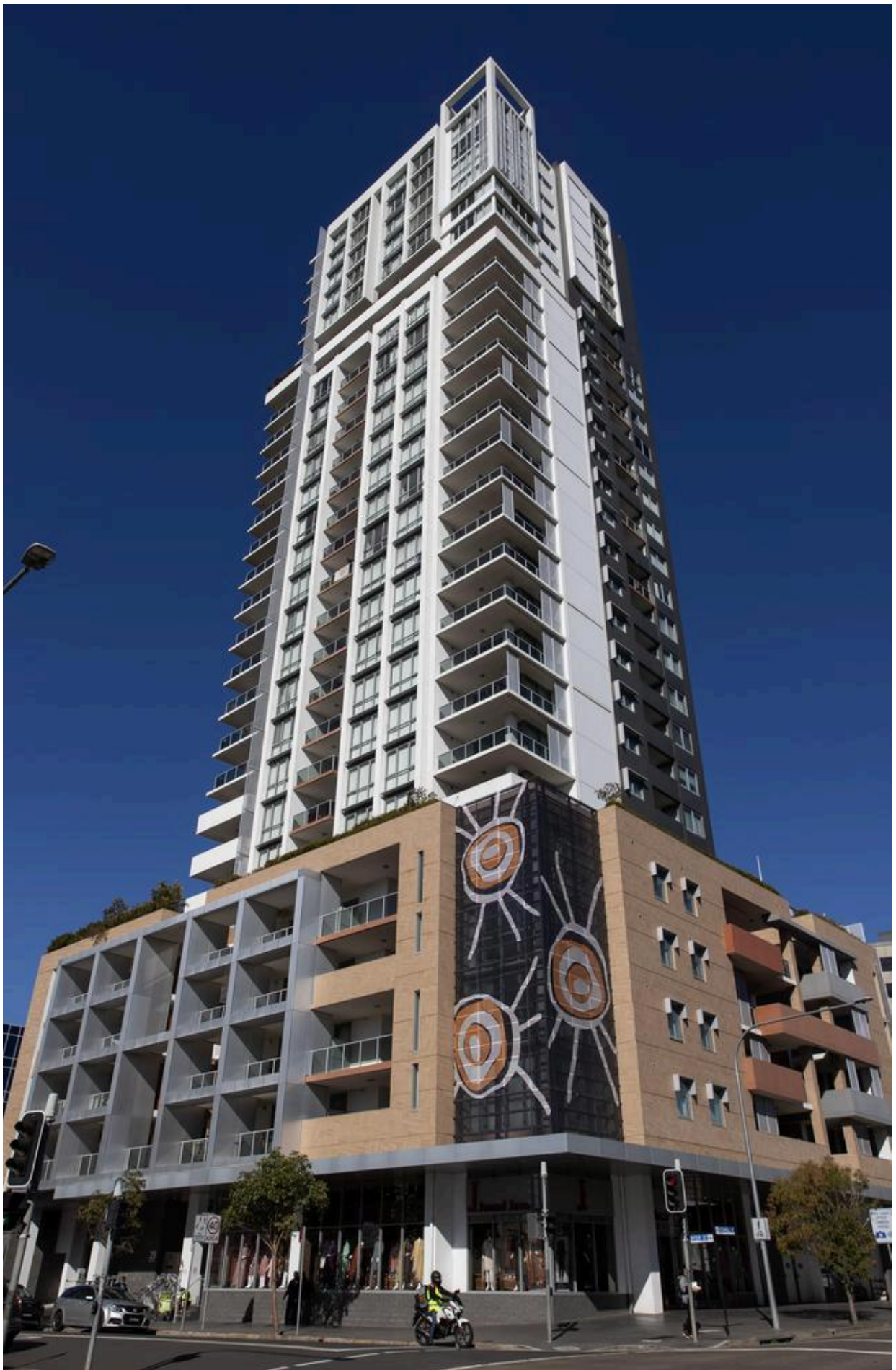
29 Hunter St, Parramatta is covered in dangerous combustible cladding. Picture: Justin Lloyd.
