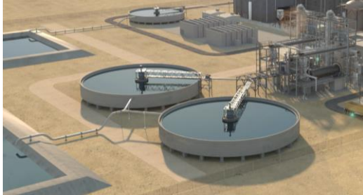
Figure 1: Thickeners at a mineral processing plant
