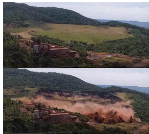
Figure 2 Brumadinho tailings dam failure in Brazil
