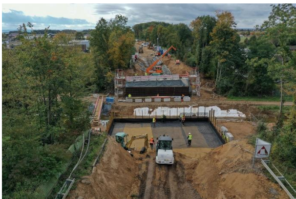
Pic 3 (2021_10_14_Heitkamp_UG_Swistal_Bruecke_L182_Bridge abutments_Copyright HEITKAMP Group):
