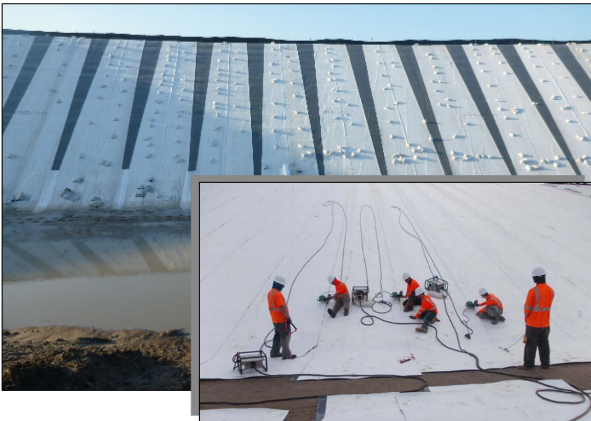
Figure 7. Photographs Showing C.W. Bill Young Reservoir Geomembrane Installation.
