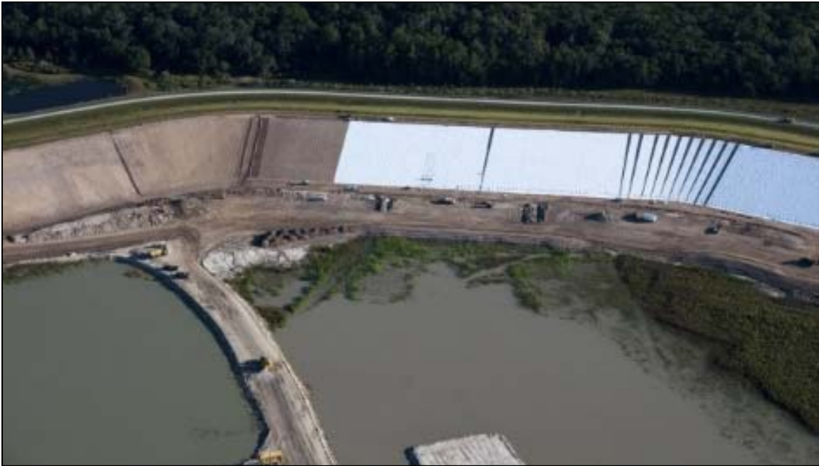
Figure 6. Aerial View of C.W. Bill Young Reservoir Geomembrane Installation
