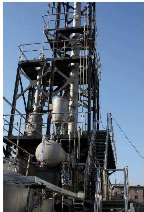
Plum's 20 tonnes per day pilot plant located in Wales, United Kingdom
