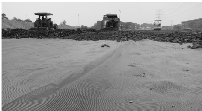
Figure 14 Placement of aggregates above Mirafi® 380a subgrade stabilisation geotextile
