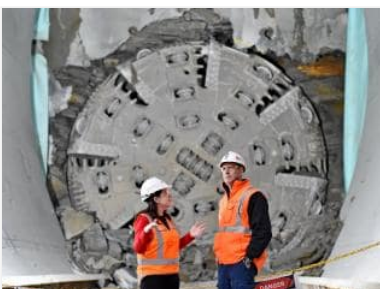
Metro tunnel breakthrough at Crows Nest
