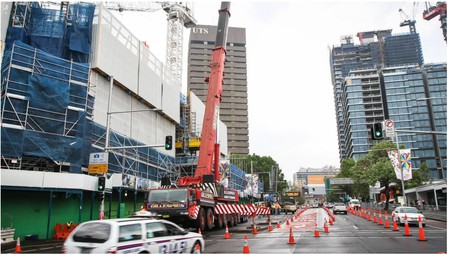
A photo of the site during construction periods.
