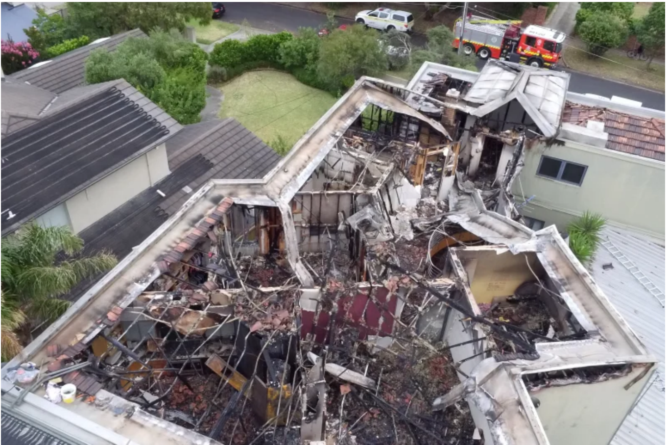
The Beaumaris home after the blaze. METROPOLITAN FIRE BRIGADE/TWITTER
