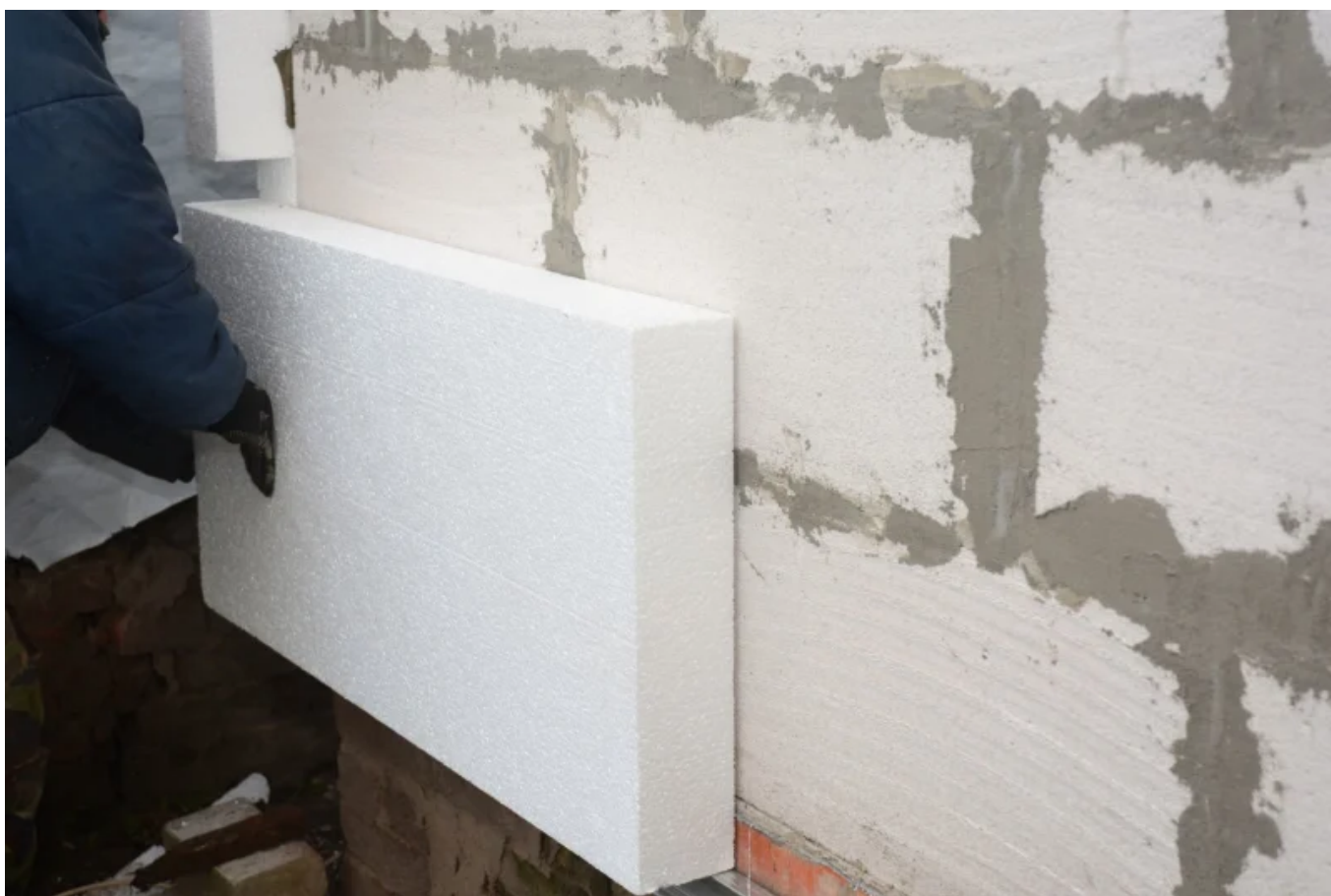
Expanded polystyrene being used in construction. EXPANDED POLYSTYRENE AUSTRALIA
