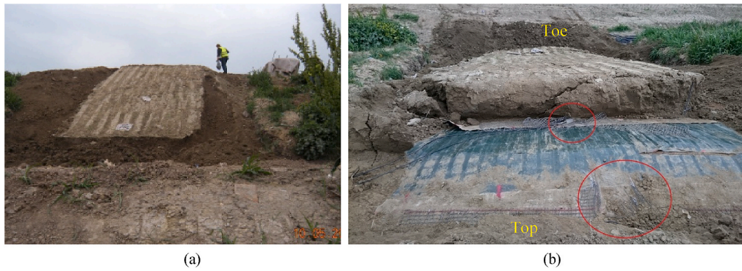
Fig. 5. (a) Slope after the removal of the soil at both sides; (b) failed slope and broken fibres (view from the top).
