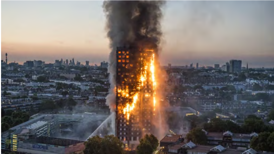
Flammable cladding fuelled London's Grenfell Tower blaze in 2017, in which 72 people died. EVENING STANDARD
