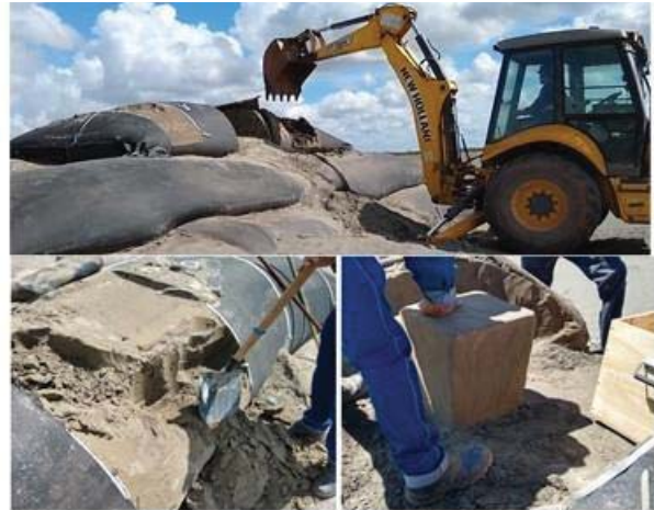
Figure 8.48. Extraction of samples from the geotextile tubes (Morais 2020).
