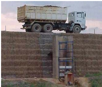
(c) Load test on one of the instrumented sections.
