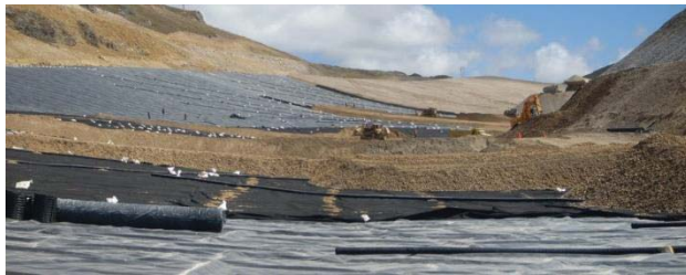
Figure 8.11: Nonwoven geotextile placed for geomembrane protection
