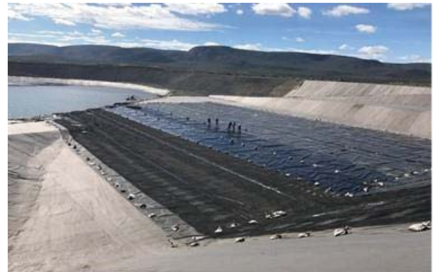
(b) Double barriers construction
