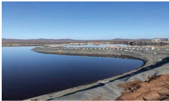
Figure 8.23. A view of vanadium Maracás dam.
