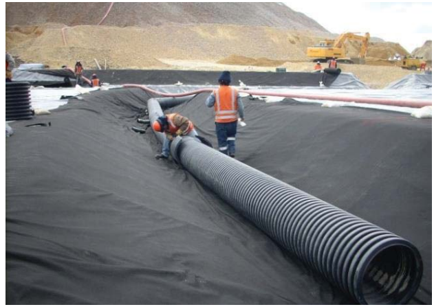
Figure 8.17: Primary collector pipe installation with geotextile for geomembrane protection
