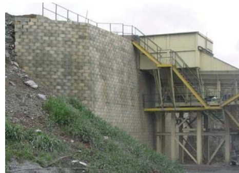
Figure 8.49. Geosynthetic reinforced wall for a crusher.
