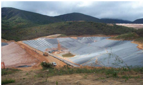
Figure 8.20. Gold tailings dams – Jacobina Dam (JYGM) – 1 st step (Sampaio, 2015).
