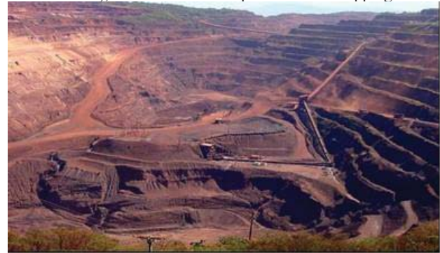
Figure 8.33 General view of Carajás mine.
