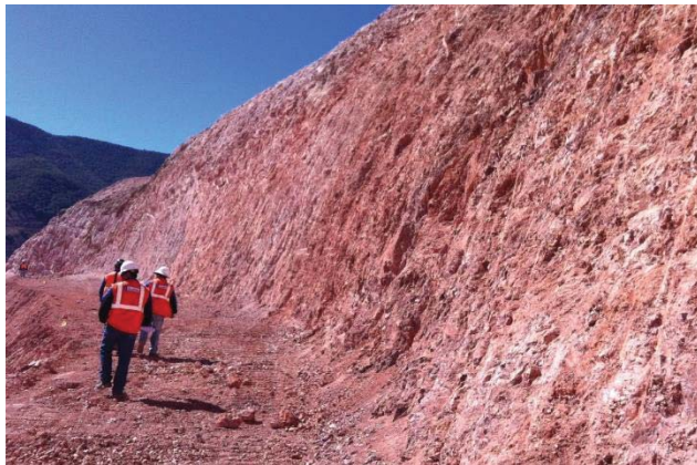
Figure 8.5: Very steep rocky slope with irregular shape after blasting
