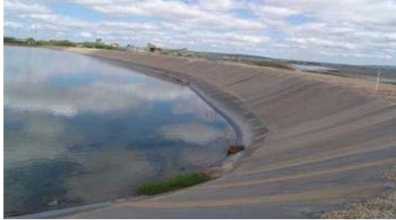
Figure 8.19. A view of Lake II (FBM) - PVC geomembrane 0.8 mm thick (Santos 2014).
