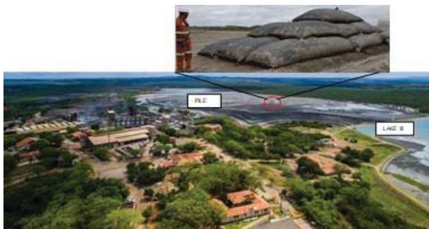
Figure 8.42. A view of Fazenda Brasileiro tailings dam (Moraes, 2020)
