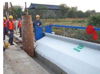
Figure 10.4 GCL/CB cut-off wall implemented in China.
