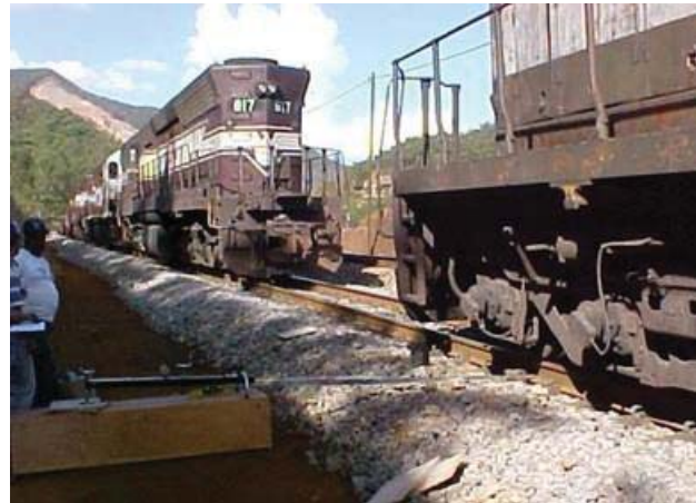
(c) Benkelman beam tests in one of the sections.
