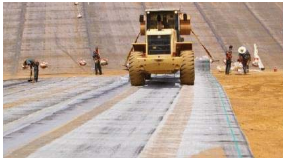
Figure 8.13: Construction equipment on bituminous geomembrane
