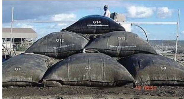
Figure 8.44. Geotextile tubes stacking – Transversal direction
