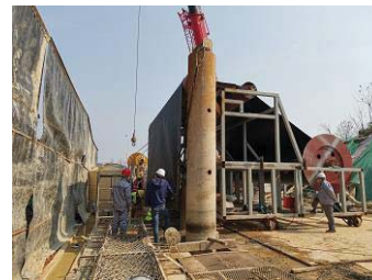
Figure 10.3 HDPE GM cut-off wall (40-m depth) in Changsha, China.
