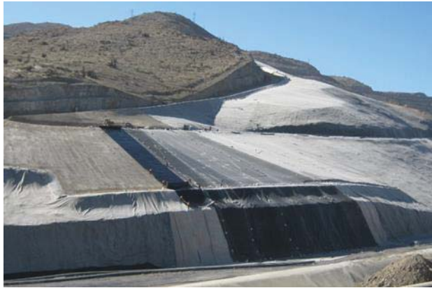
Figure 8.8: Complex geomembrane and GCL liner installation on very difficult terrain
