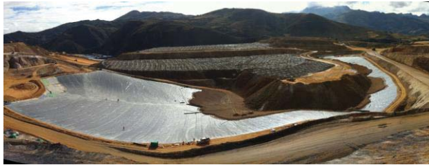
Figure 8.1: Heap leach pad (gold) in South America
