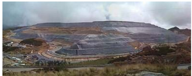
Figure 8.18: Gold heap leach pad in Peru covered almost entirely with raincoats.
