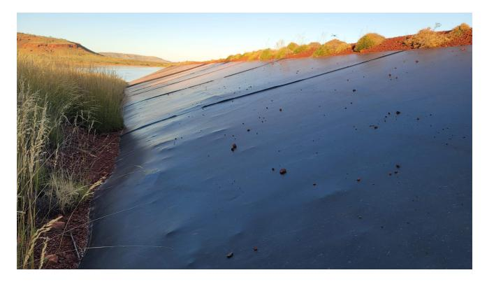
The situation is exacerbated by the presence of underlying rocks and aggregate, which can exert point loads on the geomembrane and promote stress cracking. The puncturing stresses imposed by angular rocks and aggregate on the geomembrane are significant in the field situation. The concern, particularly with HDPE, is not whether the geomembrane is punctured but rather whether it is stressed sufficiently to induce stress cracking in the longer term (see Photo 2).
