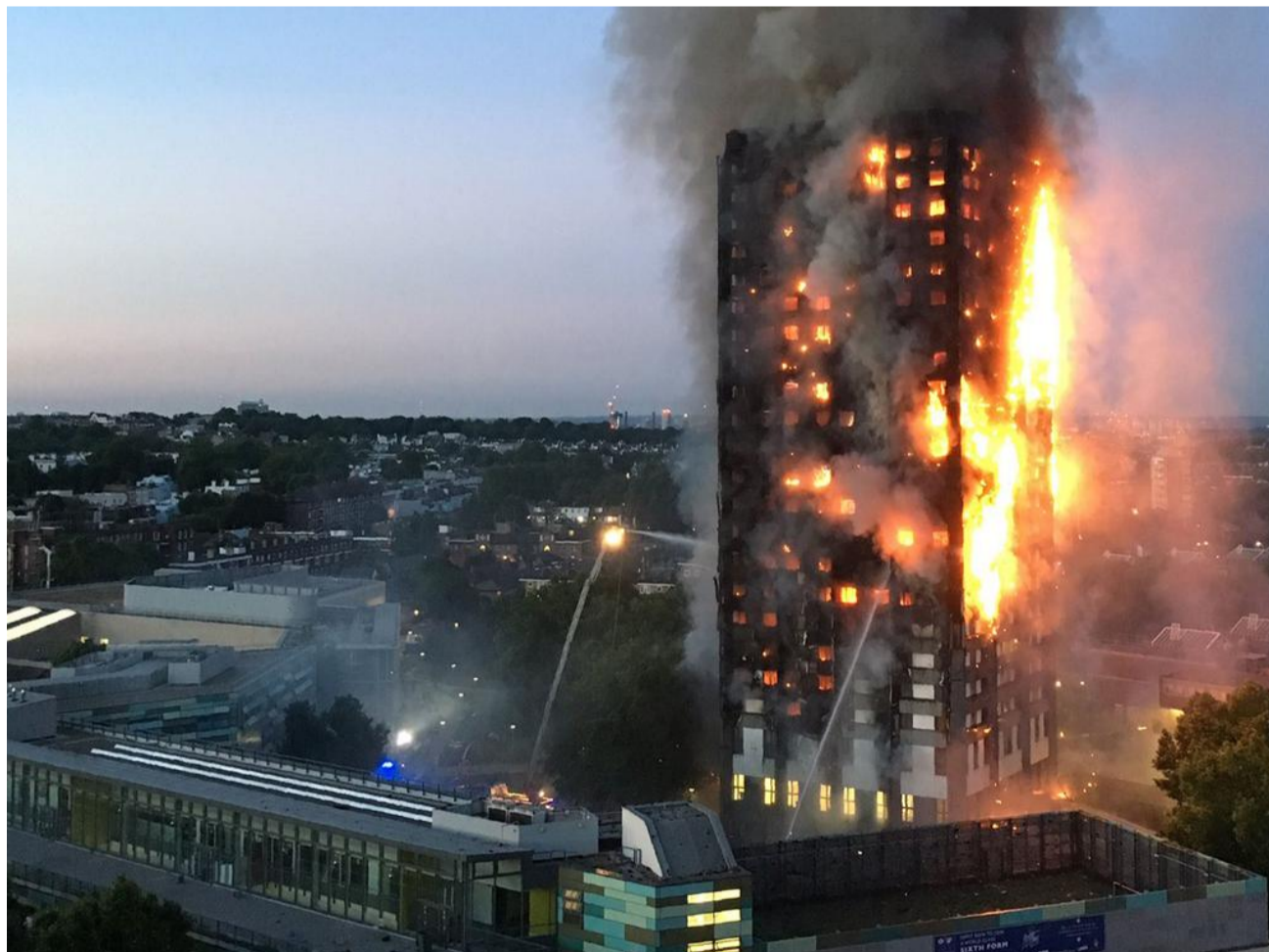
The Grenfell fire in London killed 72 people and sparked concerns around the globe about flammable cladding. Picture: Natalie Oxford /
