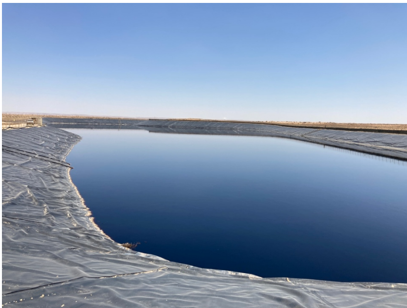
Picture of the surveyed facility.
