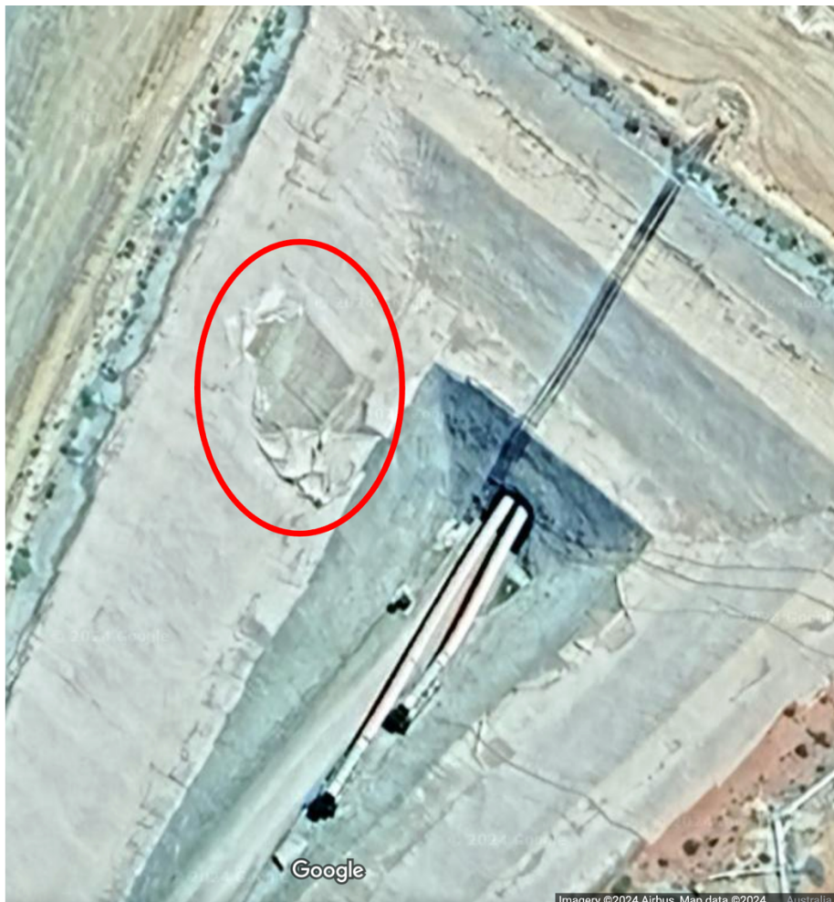
Figure 1. Shows the Tiltex surface barrier failure (in red) on the slope of the portal of the Havieron gold-copper mine in WA. [Google Maps link here ]
