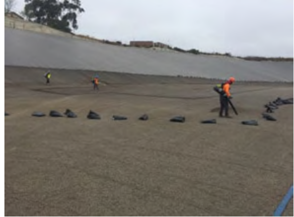
Figure 4. Cleaning existing AC subgrade prior to floating cover.
