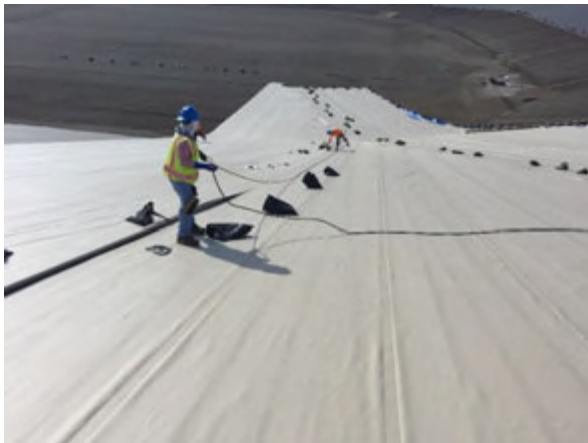
Figure 5. Floating cover panel seaming progress.
