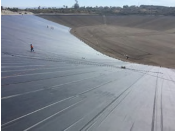
Figure 3. Chafer panel installation progress.
