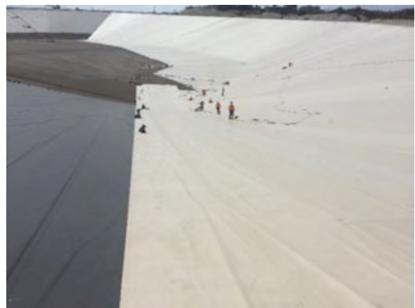
Figure 8. Floating cover and rainwater collection trough progress.
