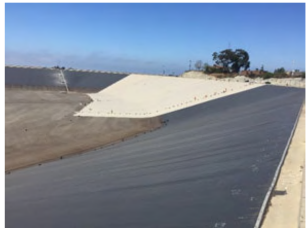
Figure 6. Floating cover fabricated panel deployment progress.
