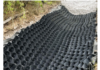
Soil stabilization can be achieved on steep embankments geosynthetic reinforcement.
